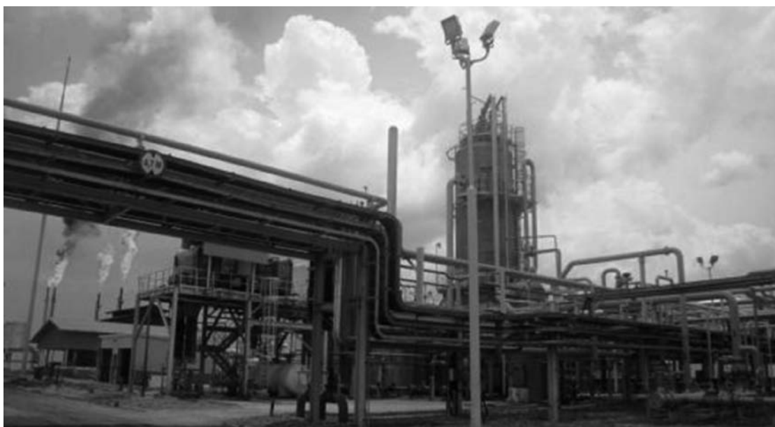
JOB Pertamina–PetroChina crude oil and gas desulphurization unit, Tuban, East Java.
