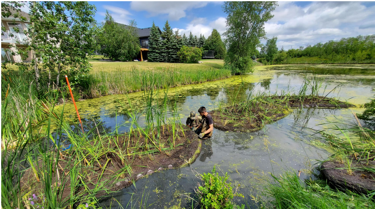
Figure 24. Floating treatment wetland deployment in the RM of East St. Paul, Manitoba
