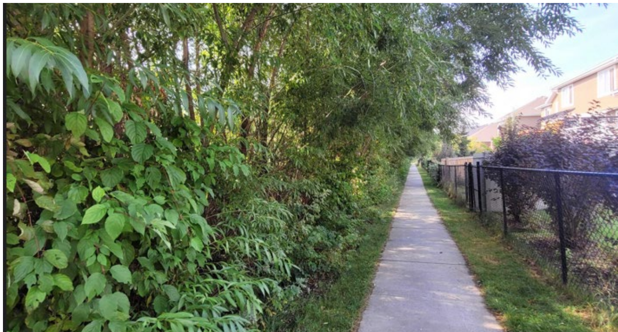
Figure 39. The well-established bioswale in the Starling subdivision in Edmonton, Alberta, in 2022
