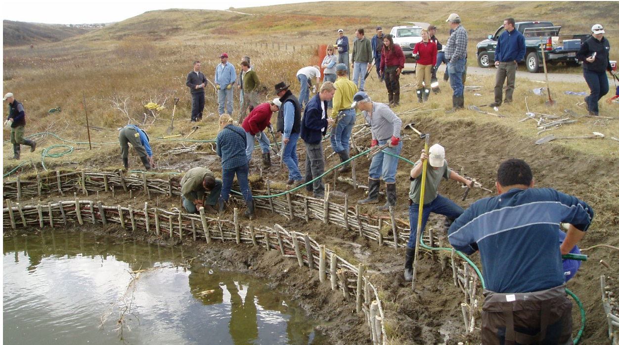
Figure 36. Wattle fencing for stream rehabilitation led by volunteers in West Nose Creek near Calgary, Alberta
