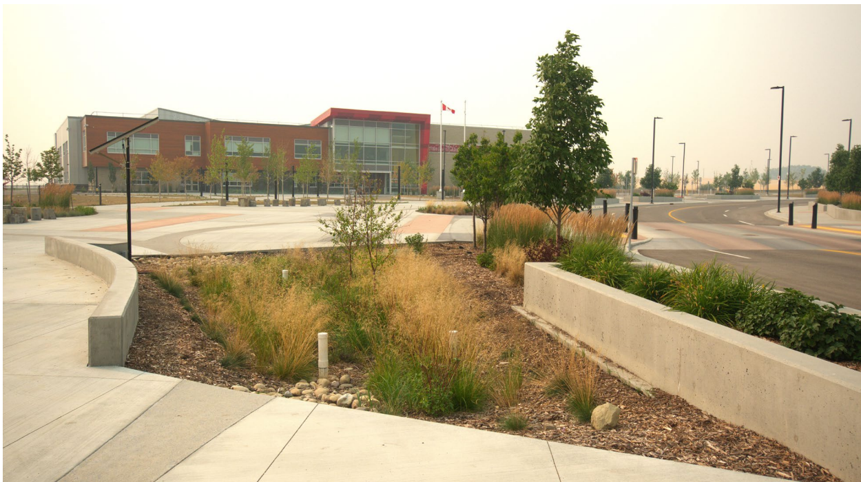
Figure 31. Drought-resilient bioretention area in Okotoks, Alberta
