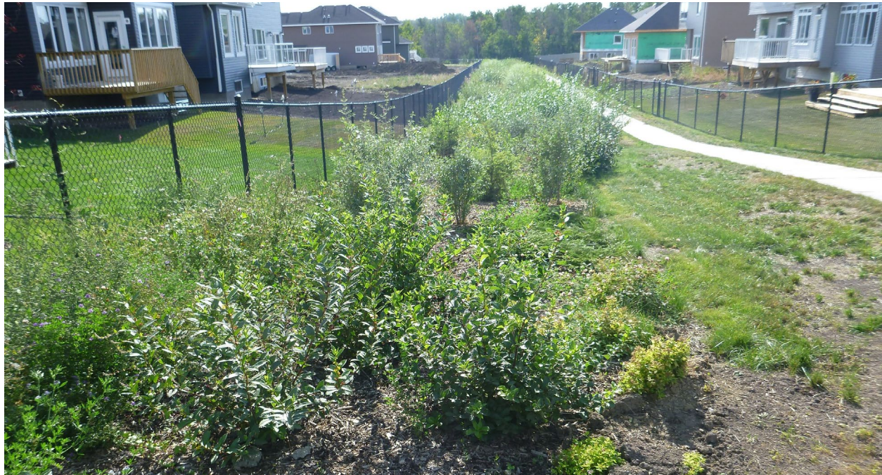
Figure 38. Bioswale in the Starling subdivision in Edmonton, Alberta, shortly after planting in 2014
