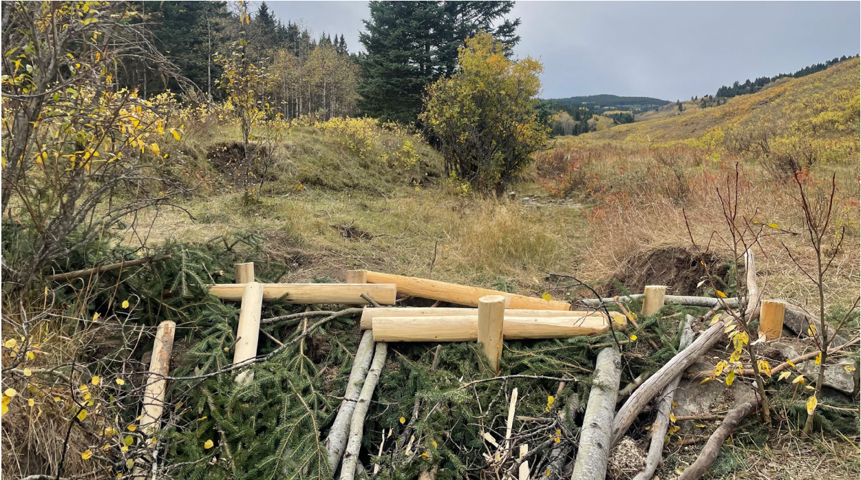
Figure 33. A beaver dam analogue on King Bolt Creek at installation (top) and the following spring (bottom).
