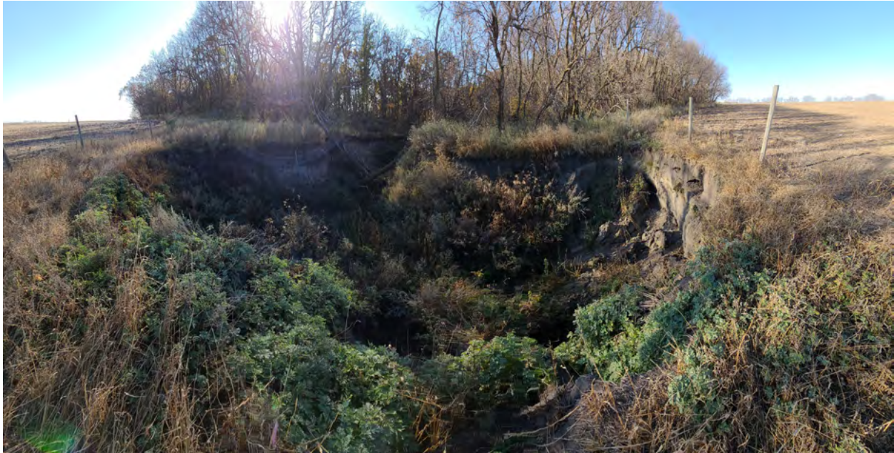
Figure 37. Previously known and highly progressed gully erosion
