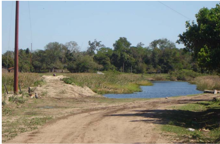
Figure 3: Wetland degradation due to increased road construction
