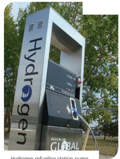
Hydrogen refueling station pump.
